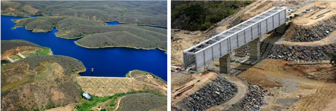
Pic. A dam in the São Francisco River Pic. An elevated channel for water transposition
